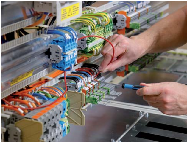
Step 5: The cable is fed in the corresponding order to the right or left to the component and can be connected again
