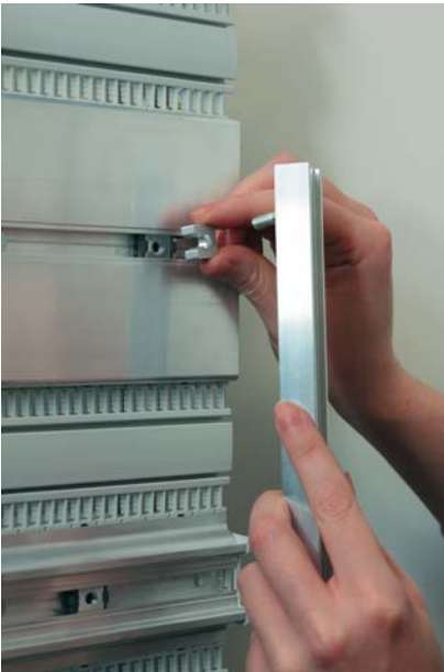
Variant 1: If DIN rail bars are built over (Type HS / HA) on assembly bars (Type MS / MA), CST 7 supports can be used to balance out the height.
