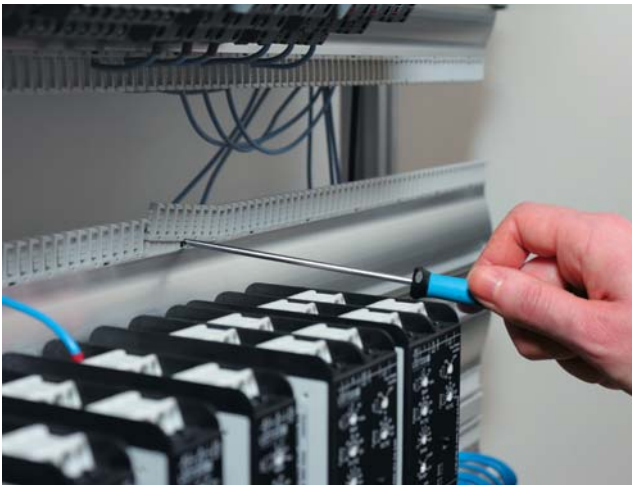
Step 1: Remove the combs with a screwdriver
